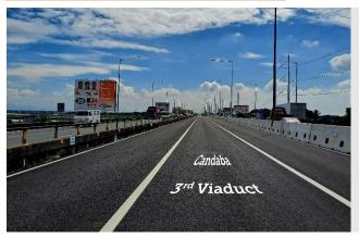
The Candaba 3<sup>rd</sup> Viaduct Project involves the construction of a 5.3-kilometer bridge built between the two existing viaducts, creating a two-bound elevated roadway. The new viaduct aims at expanding the Candaba Viaduct into a three-lane per bound roadway with wide inner and outer shoulders.
